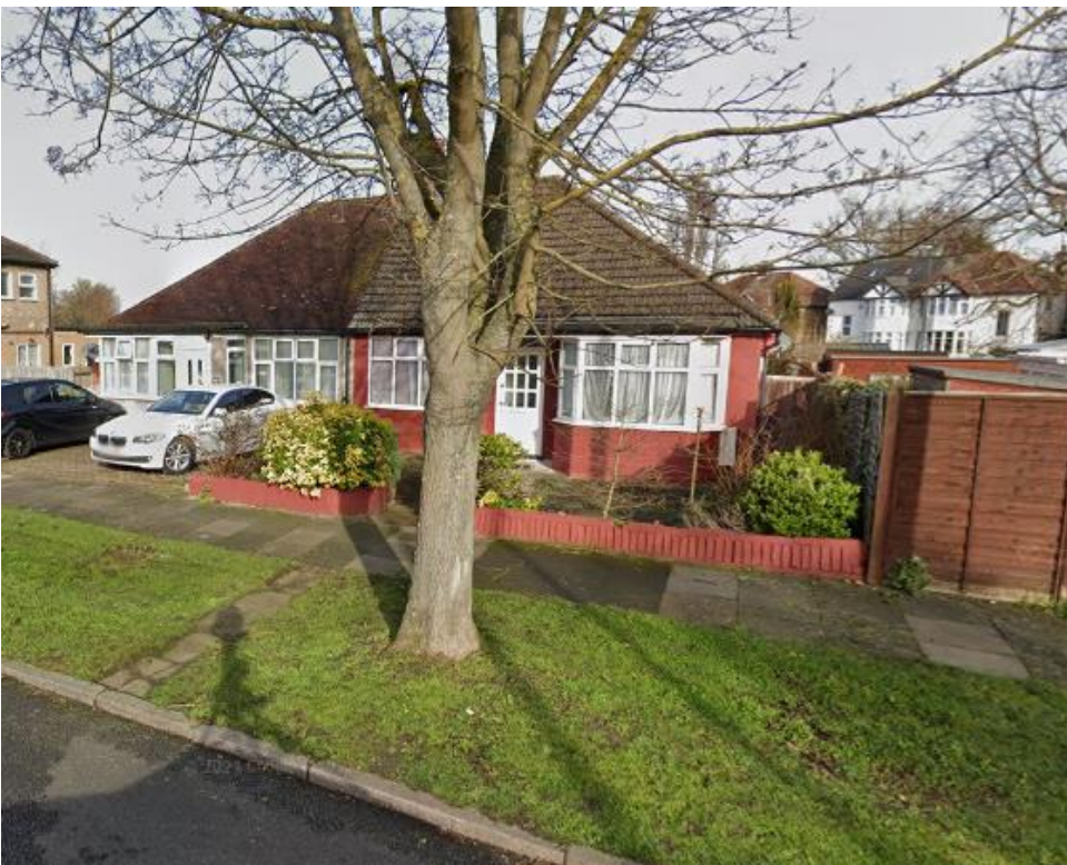
View of 42 and 42A Somervell Road:
